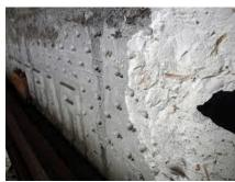
**ANSWER:** Pyrobar is a fire resistant gypsum-based product (manufactured by US Gypsum) used in construction of schools, commercial buildings, hospitals, apartment buildings and residential properties between 1903 and the 1960's. Pyrobar is white or light gray in color and was made in light-weight blocks secured together by mortar which is stacked upon one another resulting in rapid wall-like construction.
