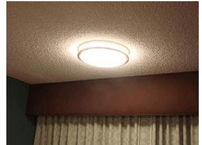
**Intact vs. Damage:** Intact (undisturbed) popcorn ceilings can be managed in-place in an Operations and Maintenance program and do not pose significant health risks. Where disturbed or debris is observed, the asbestos containing coatings may be repaired or removed and surface contamination properly cleaned up. Disturbance is often caused by:
