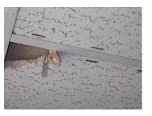
**AET's Experience:** Frequently red or pink-back ceiling tiles contain asbestos. This fact was confirmed on this survey where the tiles were found to contain 5% Chrysotile asbestos. The remainder of the ceiling tiles in the building did not contain asbestos. The specific locations of red-back ceiling tiles were identified/quantified and a thorough inspection for suspect replacement tiles performed on all adjacent floors.
