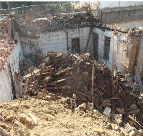
5. The wood superstructure was then removed and the wood stacked separately from the bricks. The wood was hauled to a landfill or reduced off site. The bricks were crushed and used as clean fill on the site.
