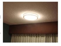
**Intact vs. Damage:** Intact (undisturbed) popcorn ceilings can be managed in-place in an Operations and Maintenance program and do not pose significant health risks. Where disturbed or debris is observed, the asbestos containing coatings may be repaired or removed and surface contamination properly cleaned up. Disturbance is often caused by:
